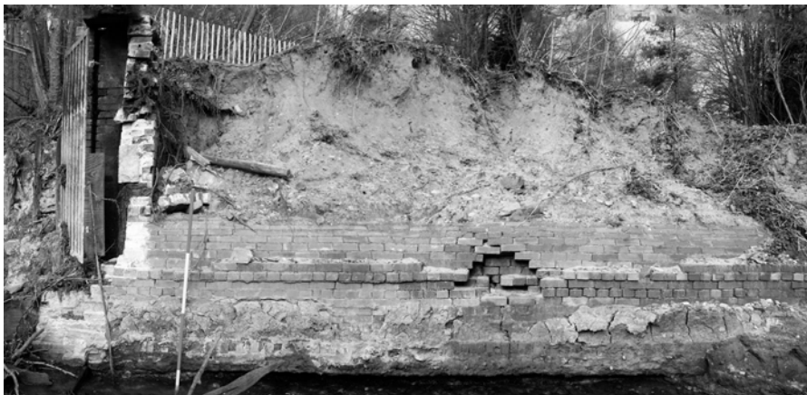
Fig 3 Photograph of west face of dam, showing the brick culvert
