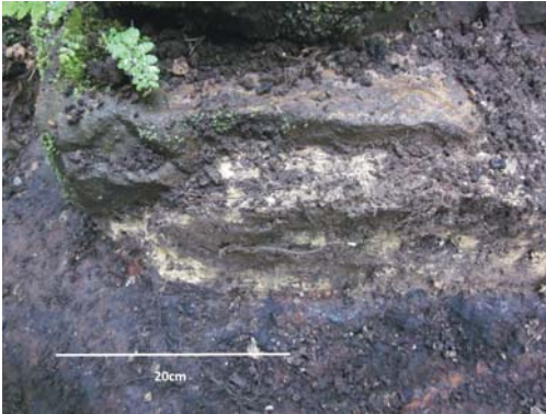
Figure 7 – Clay used to bed blocks of siderite at base of wall
