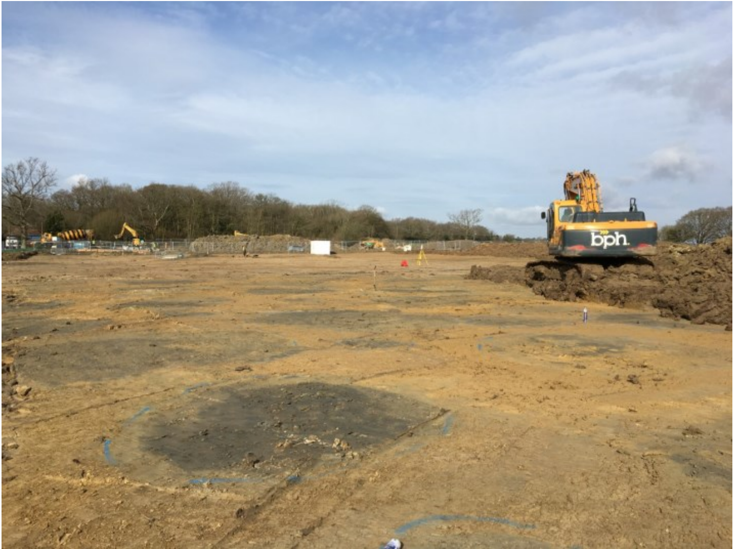
Once the ground is stripped back the minepits show as blue-grey stains
