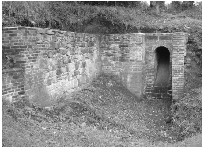
The recently consolidated masonry of the boring mill wheel pit at Ashburnham
