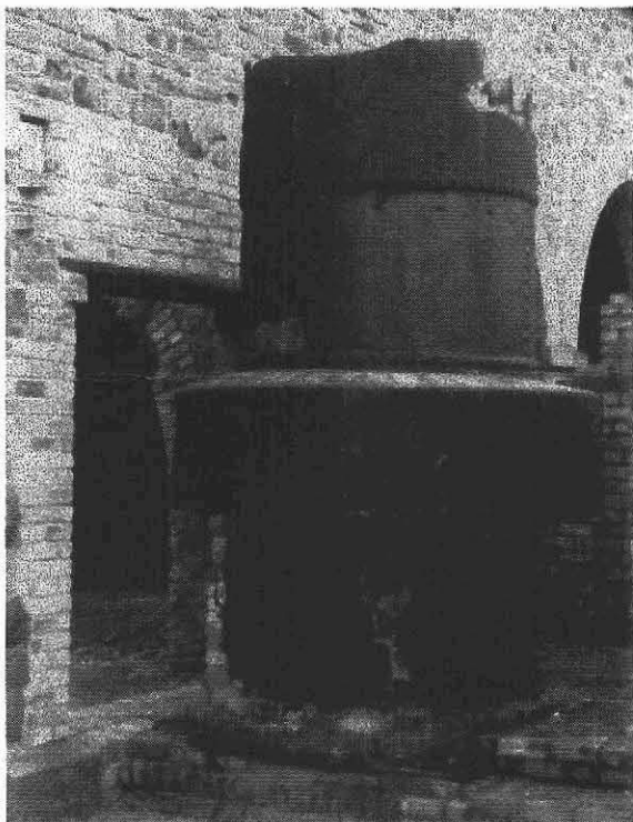
Fig 5 Gilchrist Rhomas' experimental converter at Blaenavon
