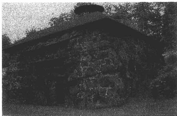
The Hogfors blast furnace, conserved with a modern roof, prior to reconstruction
