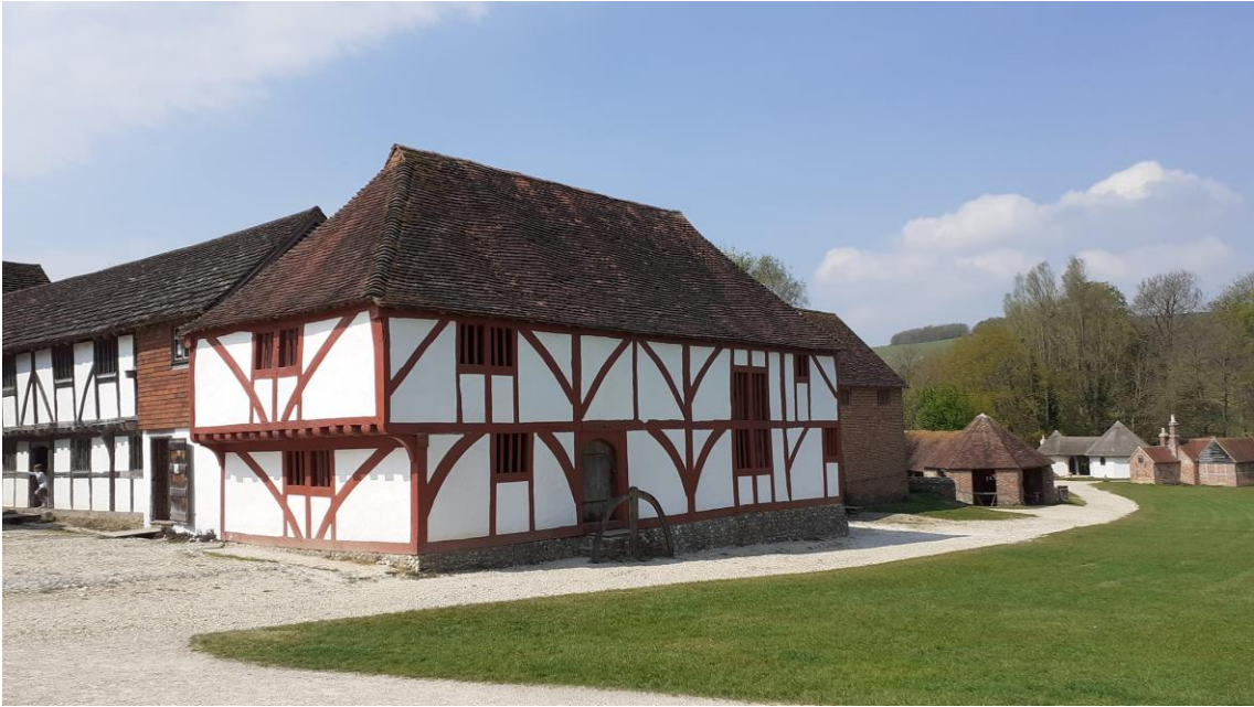
Figure 3.29 – A four bay medieval hall house from North Cray, Kent, now reconstructed at the Weald and Downland Museum. This example dates to c. 15th century and is of a similar configuration to the Brook Lane house with a central open hall and rooms at either end. Author's image
