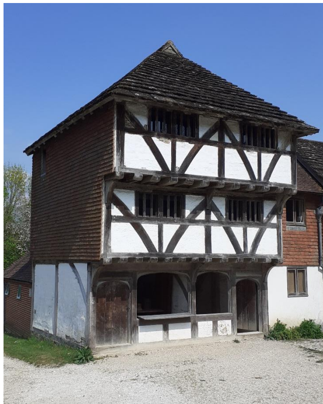
Figure 3.5 – Medieval building from Middle Street in Horsham, believed to date to the late 15 th century. It is thought that it was originally a pair of shops, although as the ground floor timbers did not survive, the current shop front is based on similar examples. The building was moved to the Weald and Downland Living Museum and reconstructed to reflect its likely original configuration (Weald and Downland Museum 2022). Author's image.
