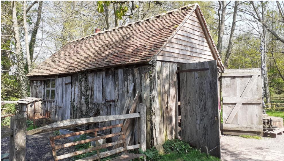
Figure 4.61 – Smithy from Southwater, West Sussex. Timber frame with roughly hewn weather boarding. (Author's image).
