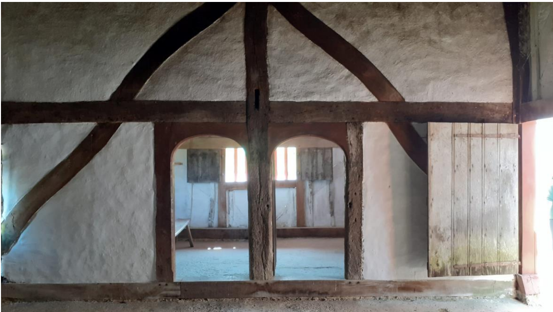
Figure 3.30 – End rooms of the open hall of the North Cray house which is divided into a buttery and pantry. The foundation evidence at Brook Lane suggested the presence separate rooms off a central hall. Author's image
