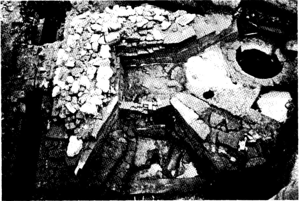
*Fig.57* Pippingford first furnace (TQ 450316). Traces of a more sophisticated drainage system than at Chingley (*fig.56*) can be seen at this early eighteenth-century gun-casting furnace. Brick channels beneath the hearth-space led to a stone drain crossing the bellows floor to discharge into the wheelpit (left foreground). (Scale: 1m.)
