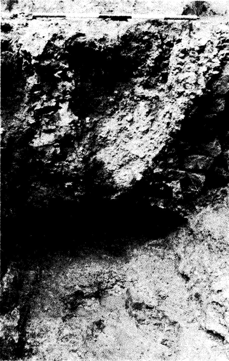
Fig.56 Chingley furnace hearth (TQ 685327): the only example so far found of substantial remains of a hearth in position in a blast furnace of the sixteenth century. The lining-stones are apparent, with the accretion of slag built up during the final campaign. A significant detail is the arch beneath the hearth, leaving a void to act as a drain (scale: 1m).
